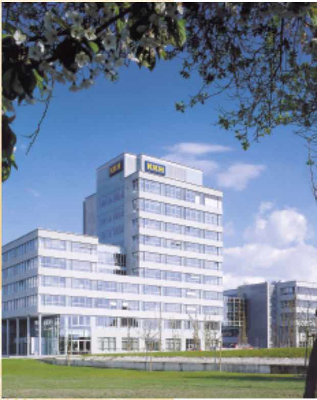
The bulding of the KKH in Hanover
